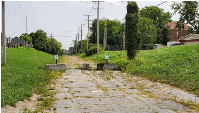
Remains of the old Hodiament Right-of-Way looking towards Taylor.
